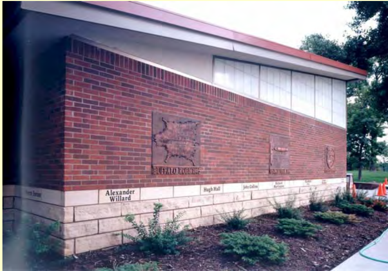
Text blocks and art blocks in masonry
