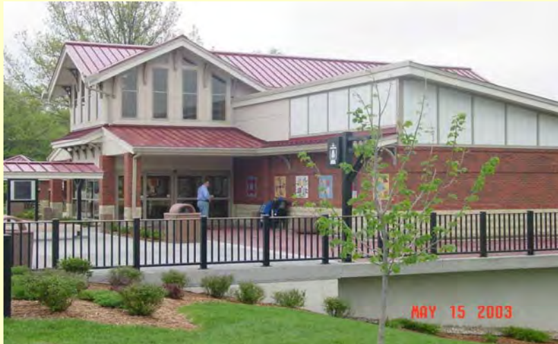
Windows and roof modified to resemble a train station
